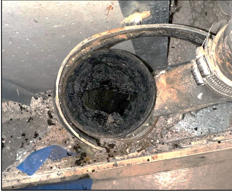
Impacted kitchen drain line in 03'
