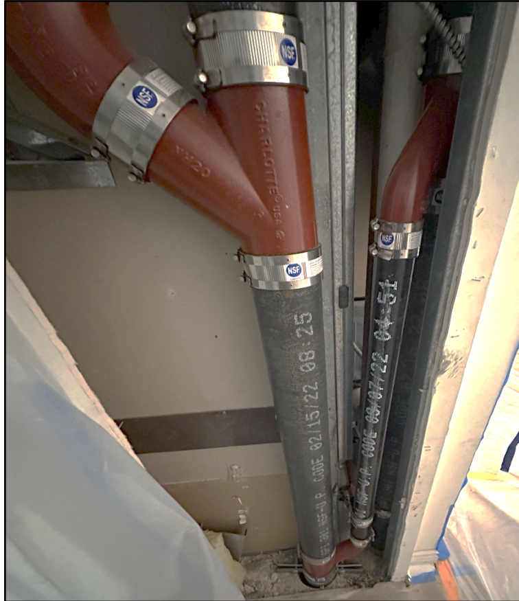
New drain line and vent 03' stack
