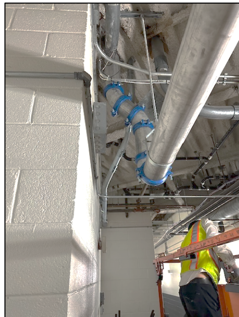
Domestic main routed through 1 st floor, up to second floor
