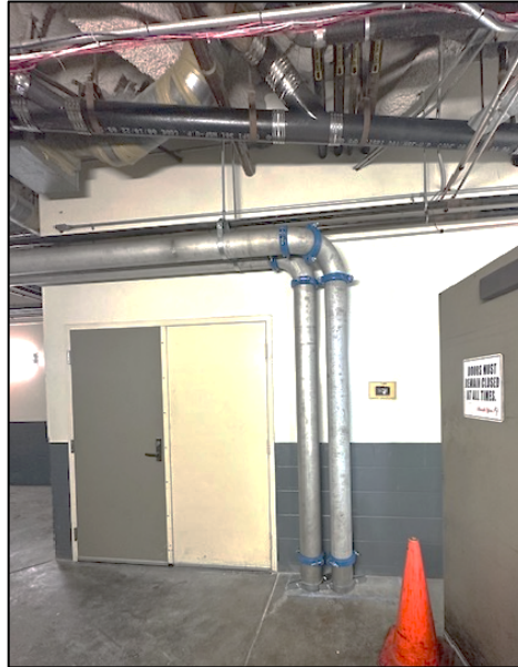
Domestic main routed through 1 st floor
